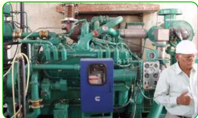
Cummins Natural Gas Engine Model Gta-1710-G duly modified for operation on 100% producer gas.
