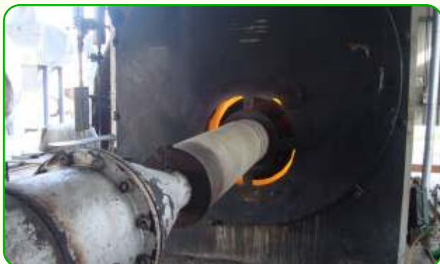
Producer gas flame replaces 4 TPH Furnace oil-fired boiler
