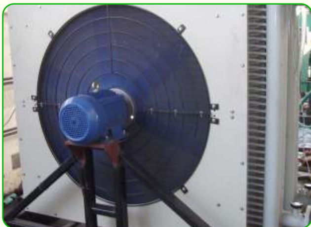
Heat recovery through remote radiator for generating hot air at around 60-70° C
