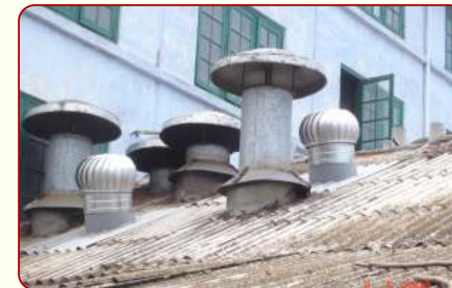
Figure 4: Use of Aero generators driven by wind in Deveshola Tea factory
