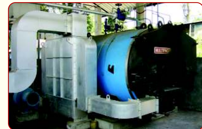
Figure 1: Thermax Wood fired Integral furnace HWG: 5th generation heating system
