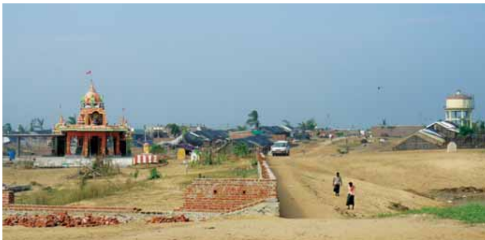
Figure 7: Village temple undamaged by Cyclone Phailin
