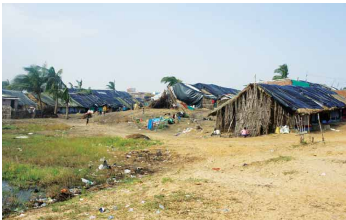
Figure 8: Damaged dwellings in Markandi village, Ganjam district
