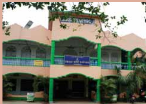
Non-IAY building at Ersama, Jagatsinghpur
