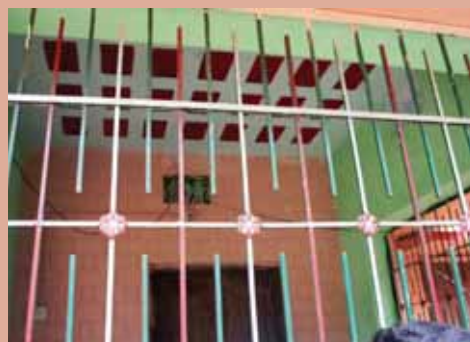
Non-IAY building at Kujang, Jagatsinghpur
