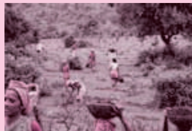
2.5.1 Women at work in SD-16P watershed project under Saltora Block
