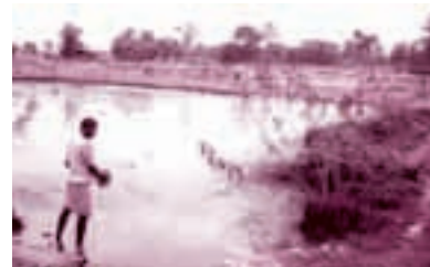
2.5.3 Construction of an earthen checkdam going on in Ranibandh Block
