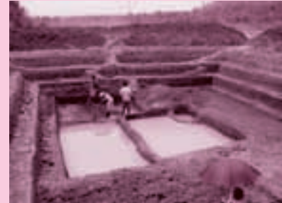
2.5.4 Construction of 5 percent model going on
