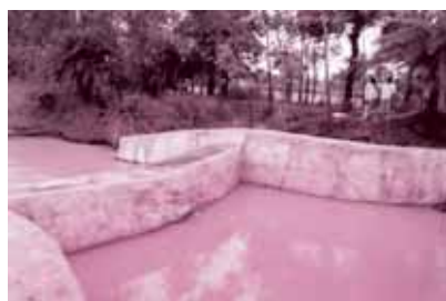
2.5.2 Checkdam constructed on a rivulet ('jore') in
