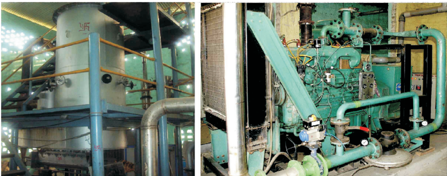
75kW Gasifier plant 100% gas engine at DESI Power site - Supplied by NETPRO
