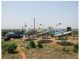
PTCs based system with 255 sq. m. area (170 PTCs each of 1.5 sq. m.) at Almond House Sweet Makers by Oorja Energy Engg. Services for heating thermic fluid required for preparation of sweets.
