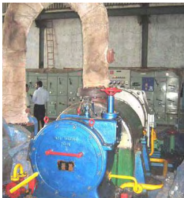
View of power turbine of a sugar mill
