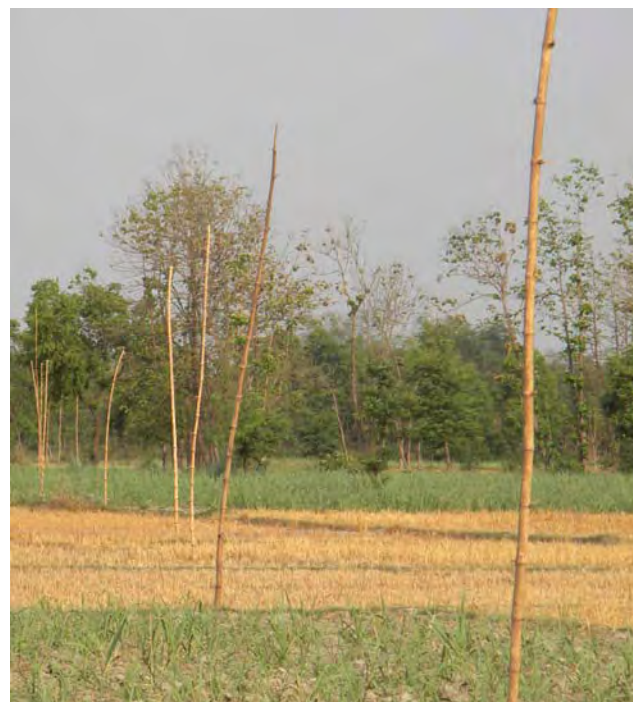
Locally available bamboo poles are used for power distribution
