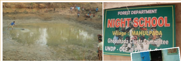
Pond renovation in progress - Sambalpur
