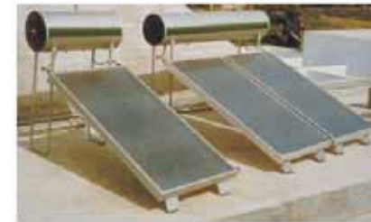
Fig6: Compact type FPC based system
