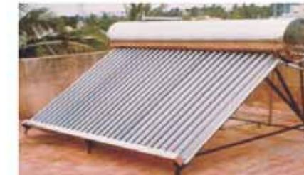
Fig7: Compact type ETC based system
