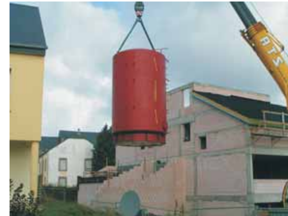
Fig11: Installation of storage tank
