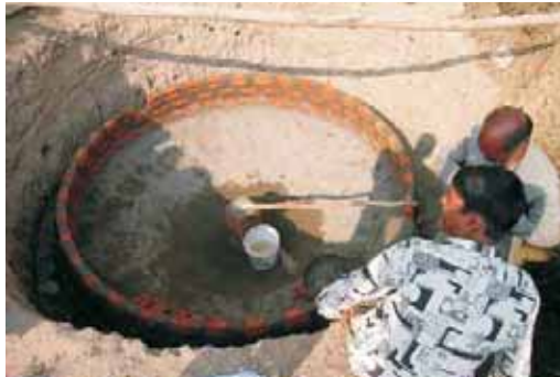
Digester Under Construction
