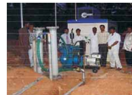
Proud Owners of Biogas Engine (10 kWh) with H 2 S Scrubber
