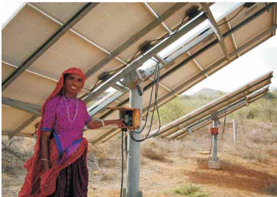
Solar Irrigation Pump
