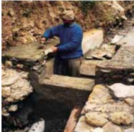
Construction of flow channel for watermill unit
