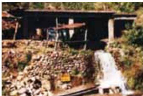
The milling house BEFORE
