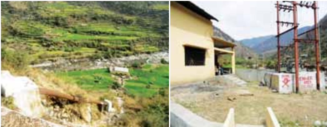
Jakhana micro hydel project, capacity 2 x 50 kW in District Tehri Garhwal of Uttarakhand
