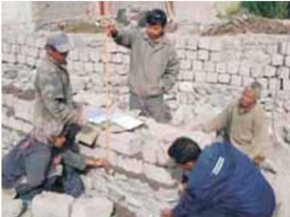
Construction of passive solar greenhouse at 14,000 feet
