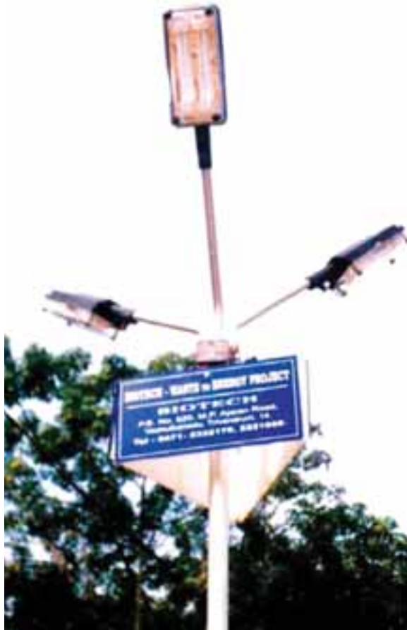
Bio-electricity lighting up streets
