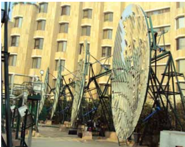
Figure 3: Dish Showing Linear Actuators at its Back
