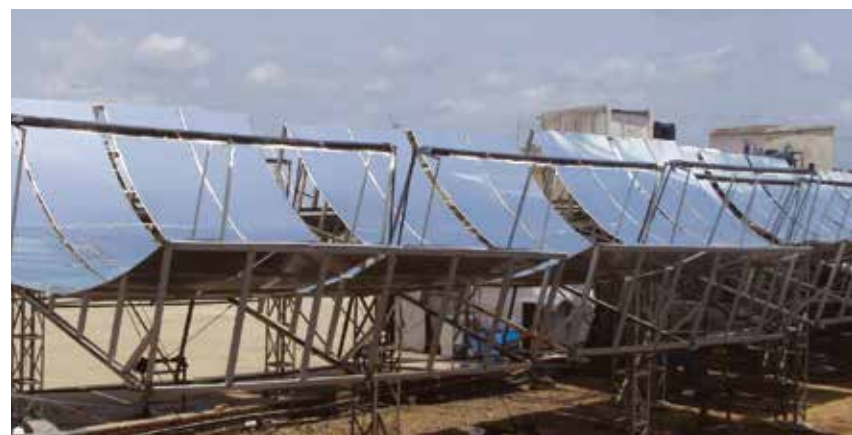
SharperSun at a surgical cotton factory using solar thermal process heat, Valsad, Gujarat
