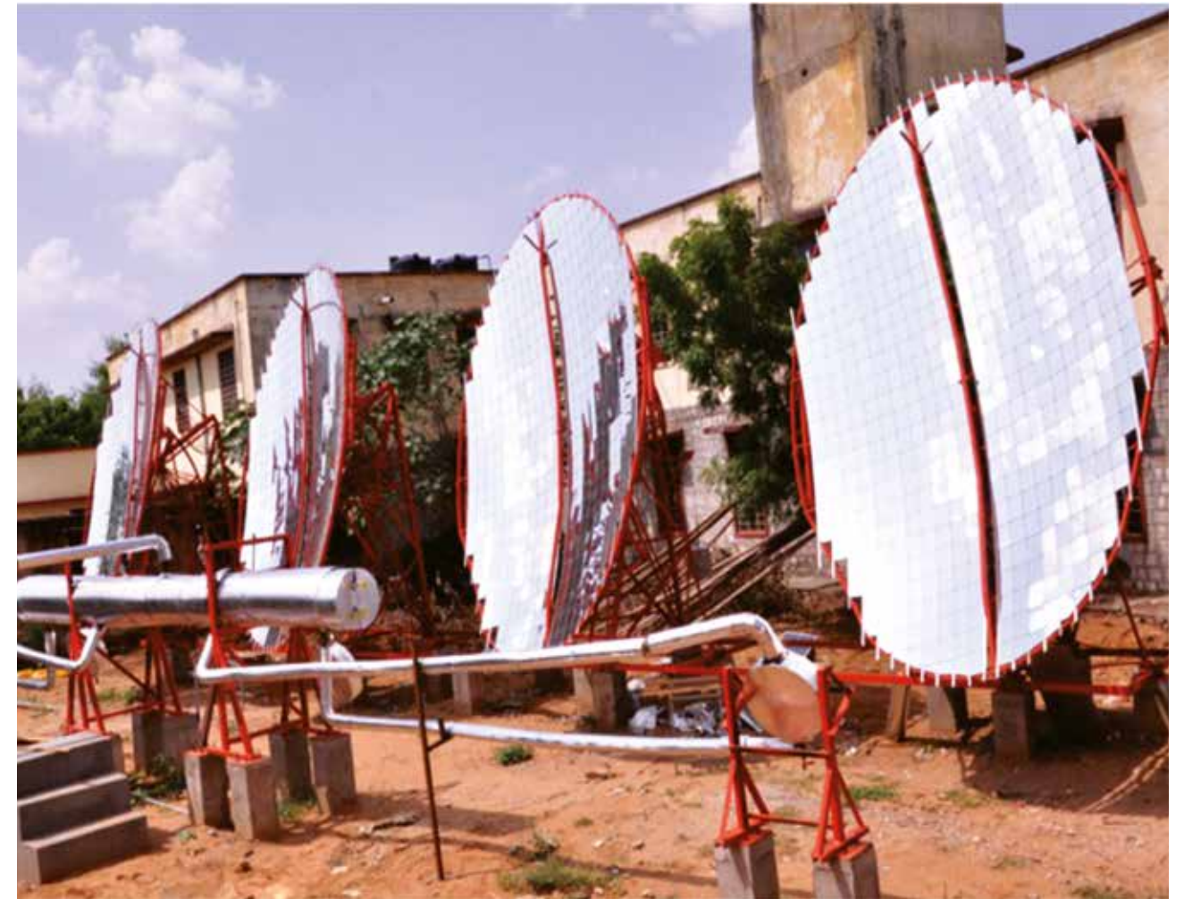
Solar steam cooking system at girls hostel of University of Rajasthan
