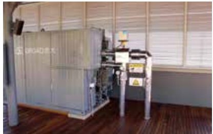
Figure 2: Double-effect absorption chiller integrated with solar collector field
