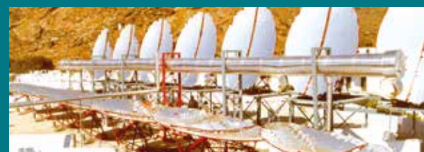
Solar Steam Cooking system for 10,000 people using Scheffler Dishes at Shantivan, Brahma Kumaris, Mount Abu.
