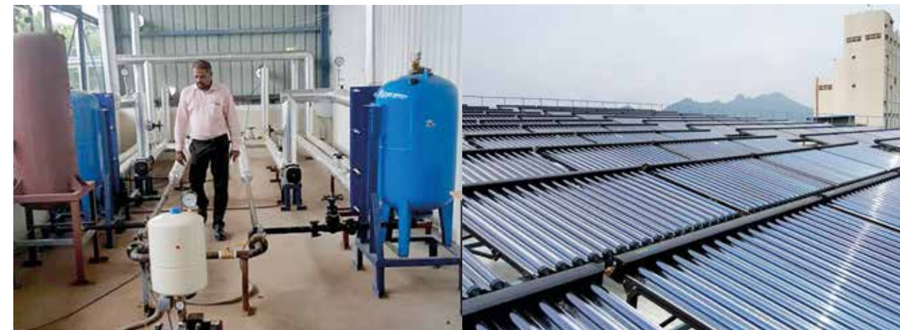
Image 1: Hatsun Agro Product Ltd Plant Uses CPC for Hot Water Feed into Boilers
