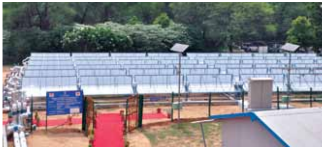
Parabolic Troughs coupled with Triple-effect Vapour Absorption Machine (100 kW Cooling Capacity)
