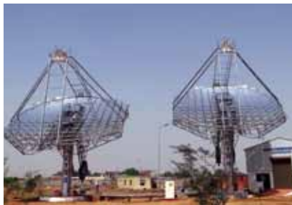
Solar Concentrator installed being used at Turbo Energy Ltd, Chennai, for space cooling
