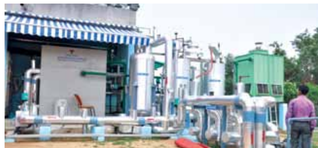
Parabolic Troughs coupled with Triple-effect Vapour Absorption Machine (100 kW Cooling Capacity)
