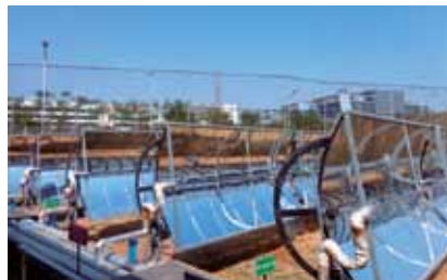
Parabolic Trough Concentrators being used for Space Cooling at Honeywell Automation Ltd, Hyderabad
