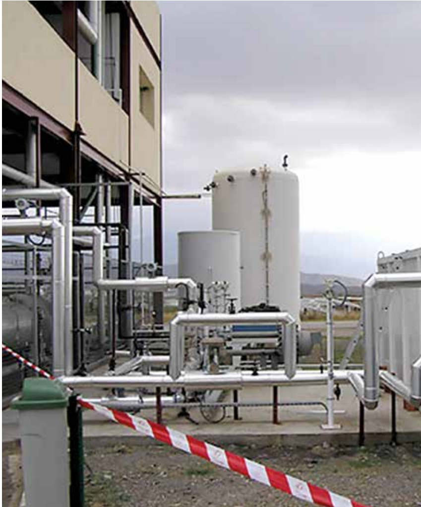
Image 3: System installed at PSA DISS (Direct Solar Steam) plant at Almeria, Spain, for PCM-based thermal storage
