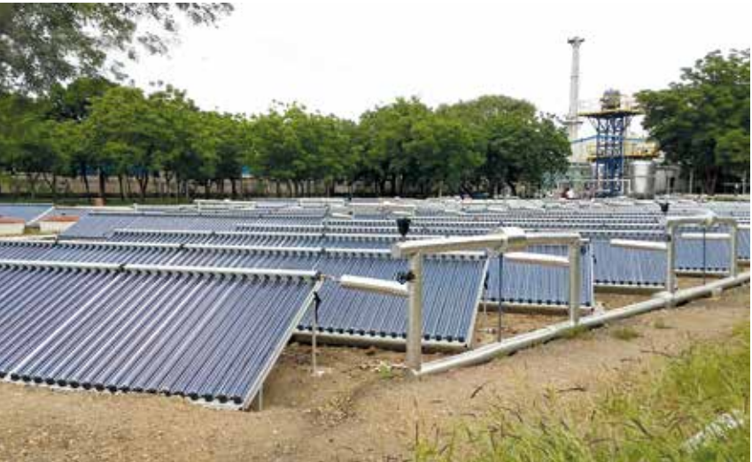
Picture 1: CPC Collectors Installed at Hindustan Unilever, Kandla, Gujarat
