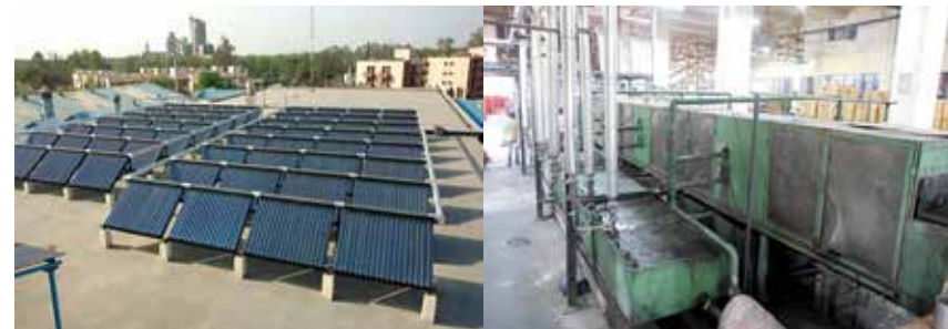
Picture 1: CPC Solar Collectors Installed at TTK Prestige for Hot Water Generation Required for Cleaning Impurities
