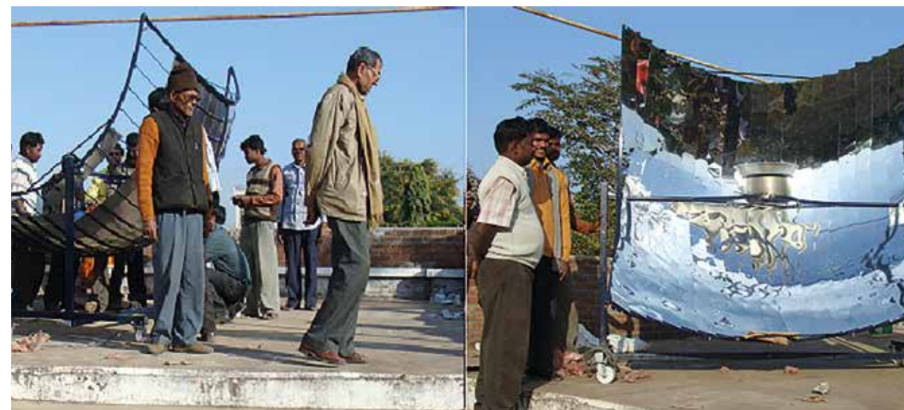
Picture 3: Tribal Workers Installing PRINCE-40 Concentrators and Cooking in Action
