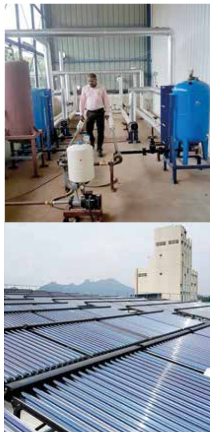
Picture 2: Hatsun Agro Product Ltd Plant Uses CPC for Hot Water Feed into Boilers
