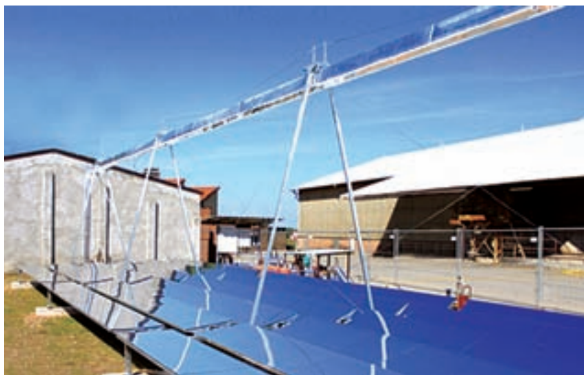
Solar process steam for brick drying at Italy installed by Soltigua, 2012
