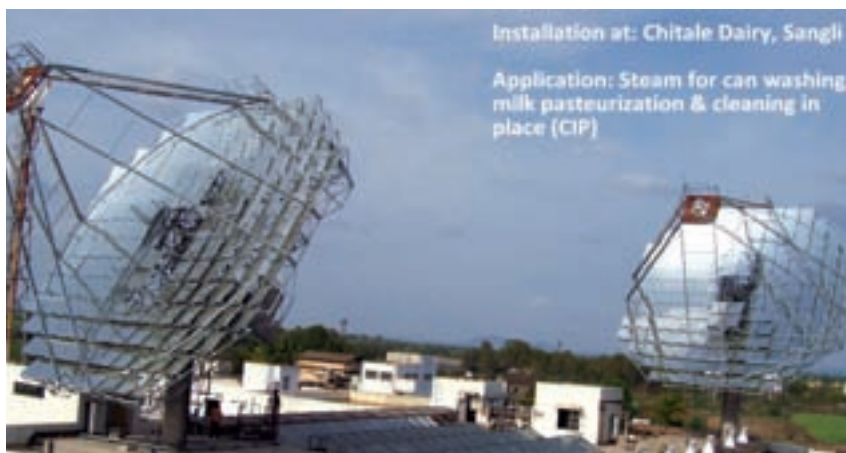
ARUN dish installed at Chitale Dairy
