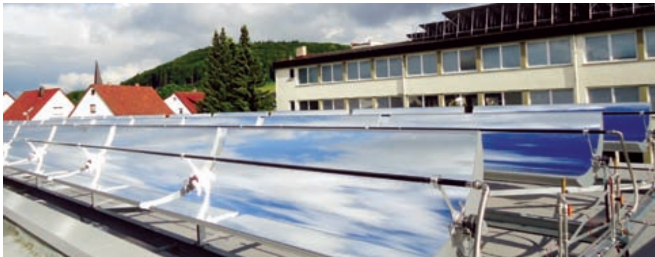
SMirro's solar steam for textile industry at Germany, 2010
