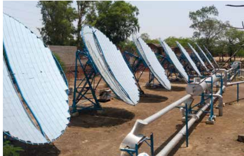
Picture 1: Concentrated solar cooking system installed at Bhandar Ghar
