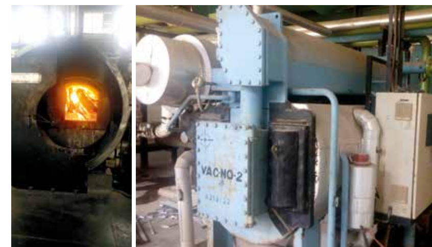
Picture 2: Boiler producing steam and vapour absorption chiller used for cooling
