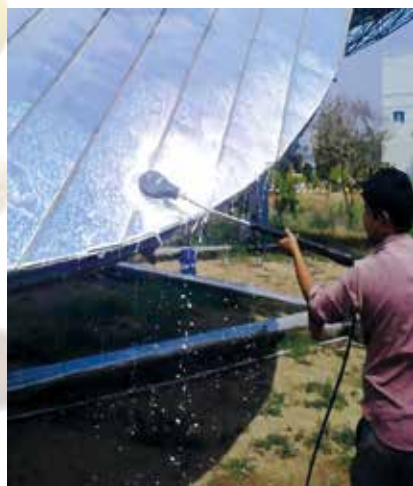
Picture 2: Cleaning of mirrors by motorized brushes
