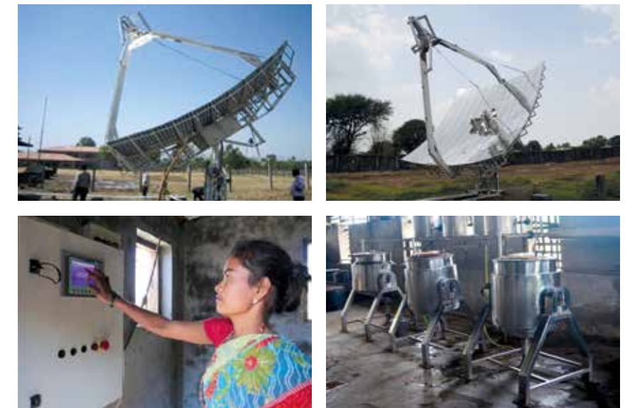
Picture 2: Concentrated solar thermal-based steam cooking system implemented by A.T.E. Enterprises Private Limited at NLC Dahanu
