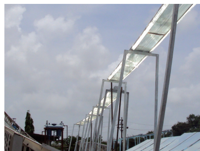
Multi-pass receiver tube used in SharperSun collector
