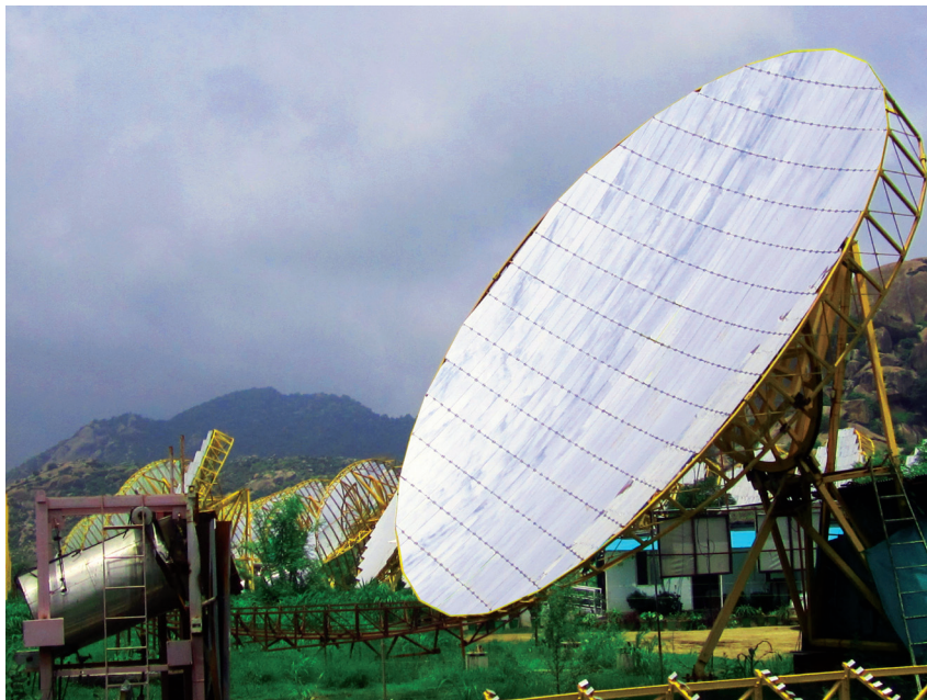
Figure 4: Fixed focus fully tracked paraboloid dish with heat storage
