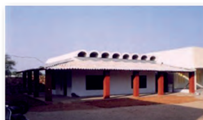
Figure I.9: DA technology jackarch & MCT roof & CSEB wall, Hyderabad
