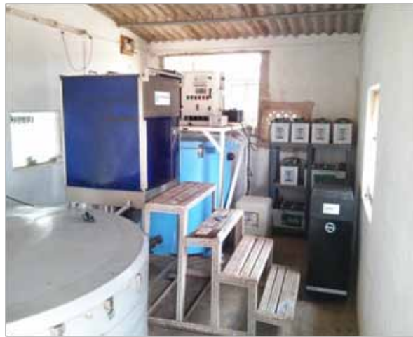
Figure 9 Solar-powered milk chiller (operates on thermal energy storage concept where solar power is used for charging the thermal battery for milk chilling)
