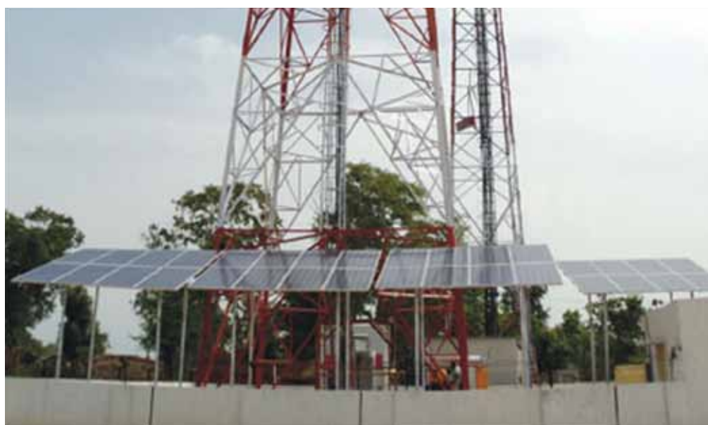
Figure 8 Solar power pack for a telecom tower
