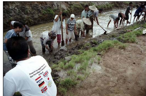
Workers clearing tsunami mud from canal in Pidie.
