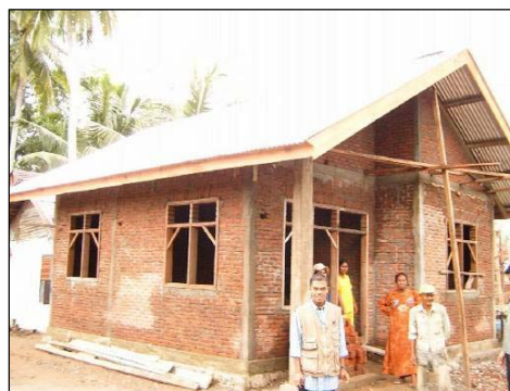
House constructed through UN-Habitat grant programme.
