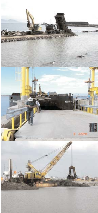
Work in progress on breakwater structure; Refurbished Ro-Ro ferry ramp; Removal of Tsunami debris from Ulee Lheue Harbour.
