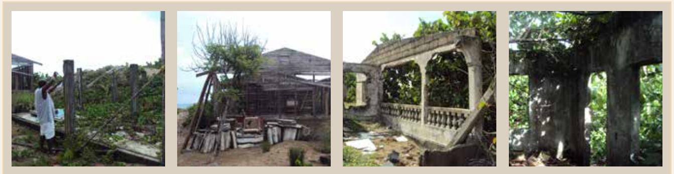
Photos of some demolitions to be done
