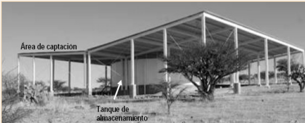
Rainwater capture by roof catchment (Anaya and Martínez, 2007)
