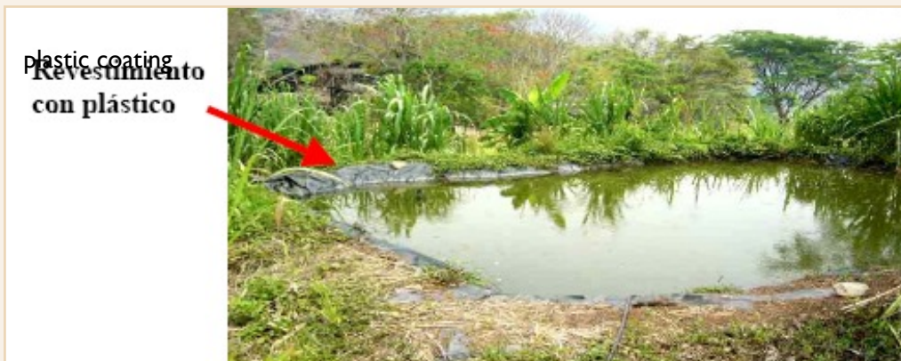
Example of a pond lined with black plastic (CATIE, 2006)
