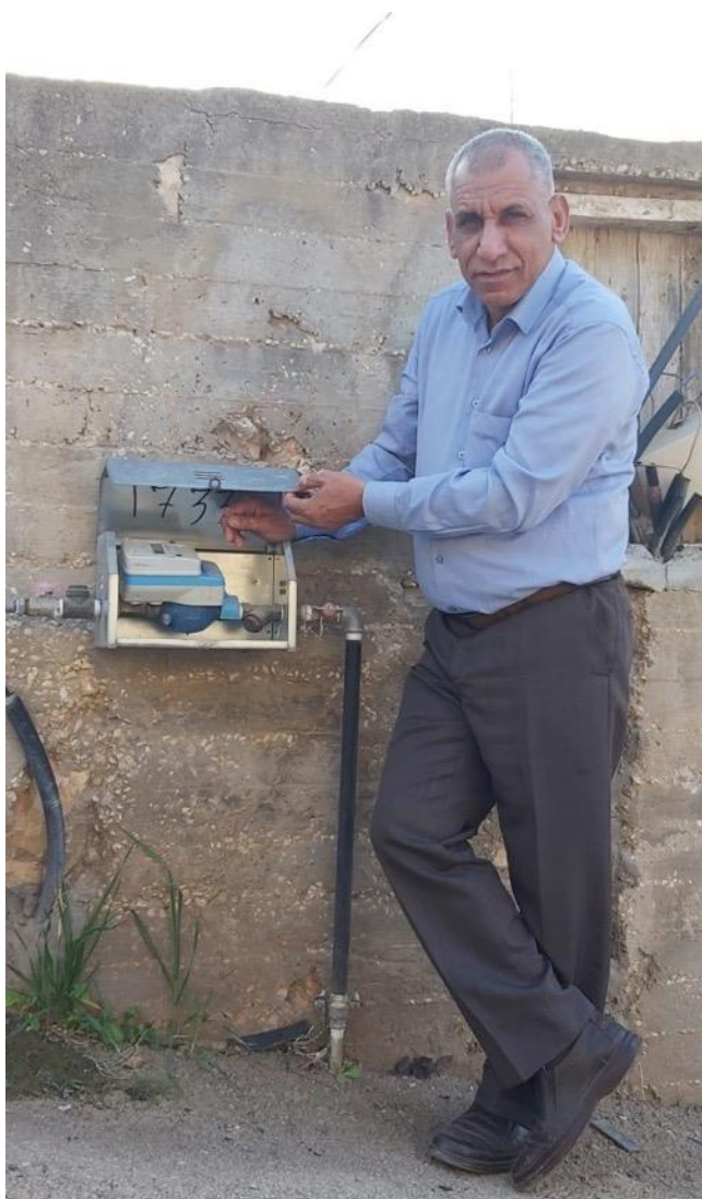
Engineer Dababat checks the water meter of a family in the Tubas district, Palestine. Thanks to a local innovation identified by the UNDP Accelerator Lab, Dababat can now fix any faulty water meter quickly and cheaply.
