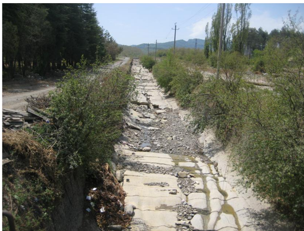
Photo 1 Concrete River channel Damage
