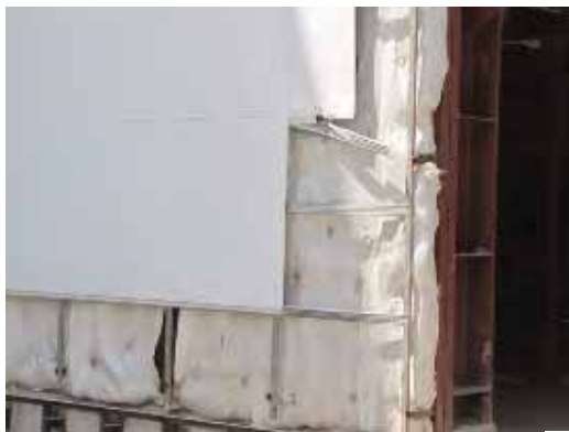
Ventilated façade, National University in Tashkent
