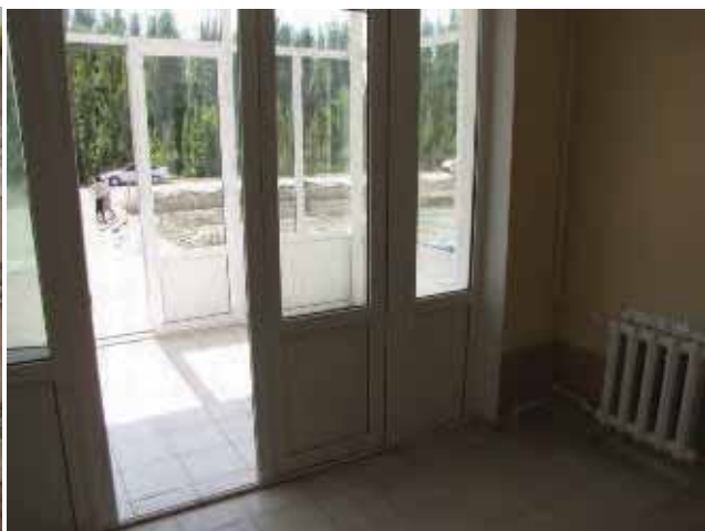
Enclosed entryway with plastic frames and sealed glass
