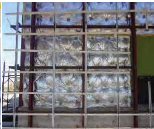
Insulation in ventilated facade. Urgench airport
