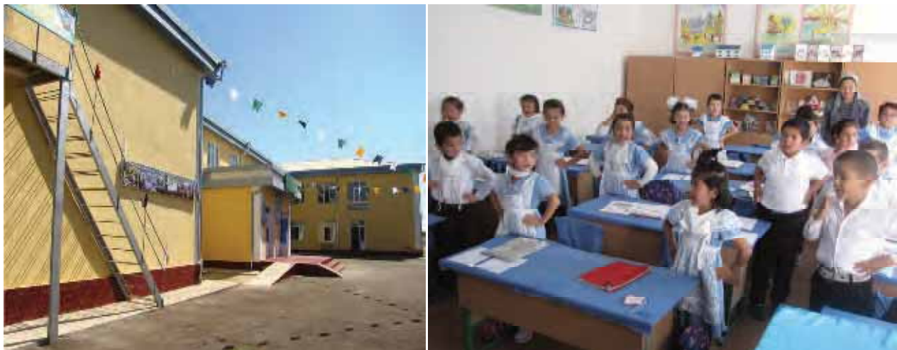
Renovated school in Karshi, Kashkadarya region. Renovations designed and implemented by the EEPB project have reduced heat energy consumption by 60 percent. Teachers note dramatically increased comfort and reduced student illnesses as well.
