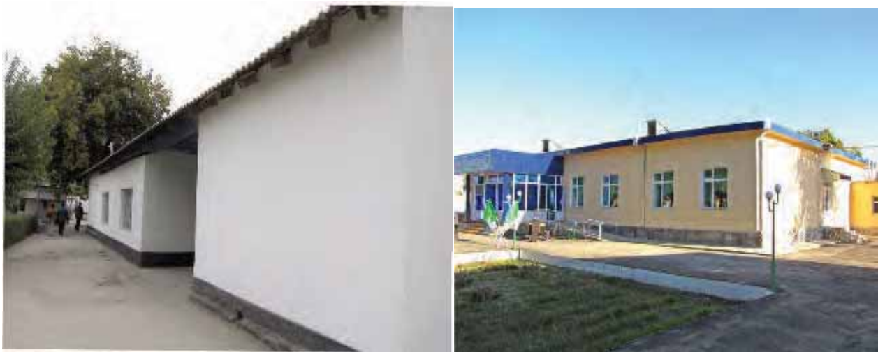
School No. 35 in Yangirabad, before and after renovation designed and implemented by the EEPB project. Heat energy consumption has been reduced by 61 percent.
