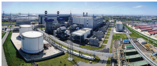
Figure 25. Adler combined heat and power station
