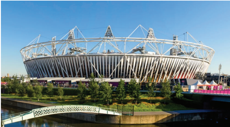
Figure 15. London 2012 Olympic Stadium (Source: David Stubbs, London 2012)
