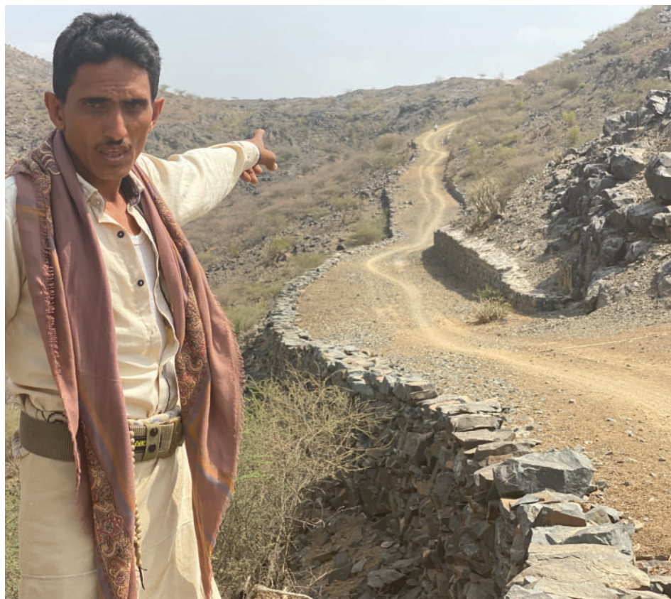
Adel pointing to the rehabilitated road in Al-Markh Valley, Bajel, Hodeida
