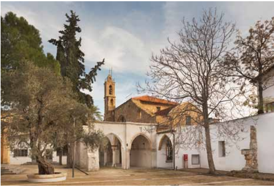
External view of the restored Armenian Church and Monastery.
