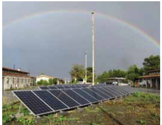
UNDP-ACT solar panel installation in the UN Protected Area.
