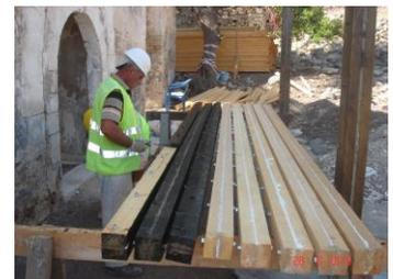
Emergency measures included: general cleaning, removal of debris and vegetation from the building and inside the yard, consolidation of deteriorated masonry in order to prevent it from further collapse, control of organic growth, excavation, permanent timber structural support, and consolidation of the walls and provision of a temporary roof to prevent rainwater infiltrations.
