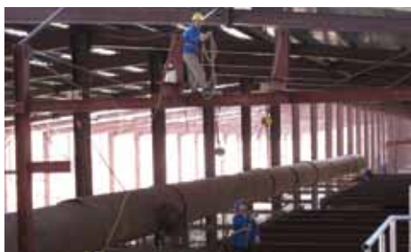
Figure 8. Installation of WHRPG Components at the Xinrong Pilot Plant
