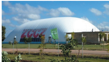
Multi-functional air dome in the Lusaka-East Multi-Facility Economic Zone used for recreational activities by workers, such as basket ball and volley ball as well as for events.
