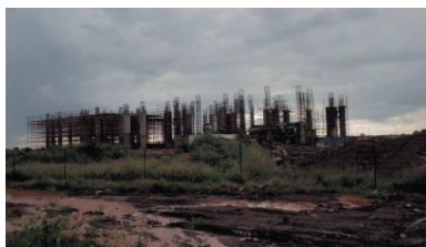
Zambian Breweries Malt Plant under construction
