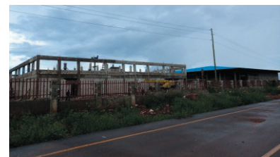
NRB Pharmaceutical plant under construction
