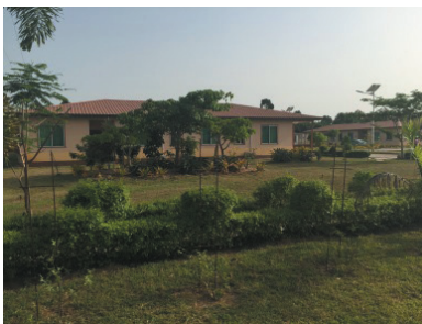
Dormitory of company managers and LFZDC personnel
