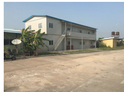
Dormitory of workers
