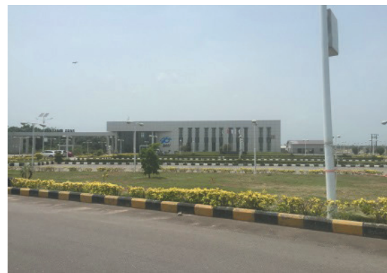
Inside the Lekki Free Zone Development Company Administrative Complex
