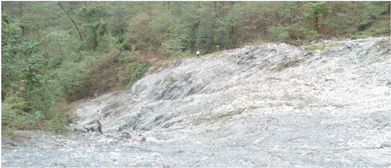
Figure 5 Initial Land Slide at the Box Cut
