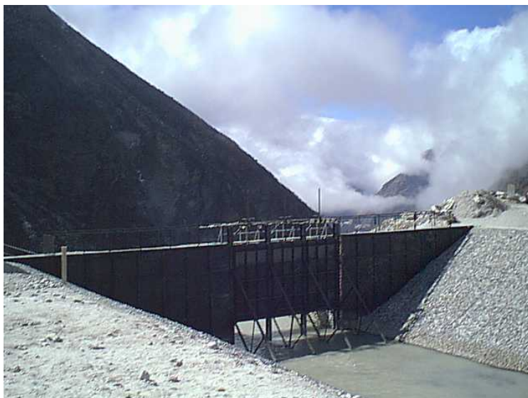
Figure 6 Excavation of the left lateral moraine of Tsho Rolpa and the installation of a permanent sluice to control outflow of the lake, succeeding the lowering of the lake level by 3m. Photo source: rolwaling.tripod.com/2k/2k-tr-fix.html
