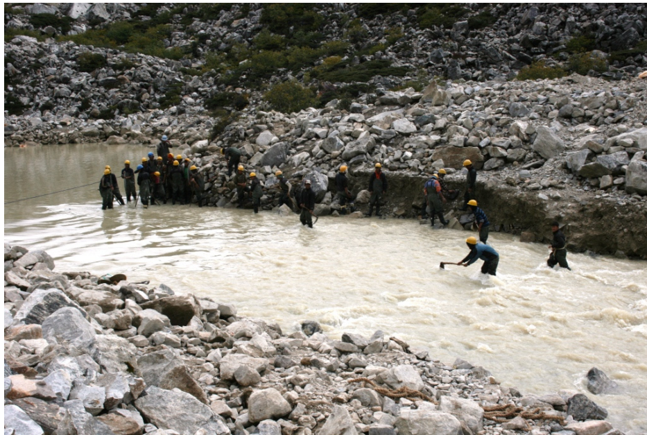
Figure 5 Excavation works in the channel between Subsidiary Lake 1 and 2: difficult working conditions in cold fast flowing water
