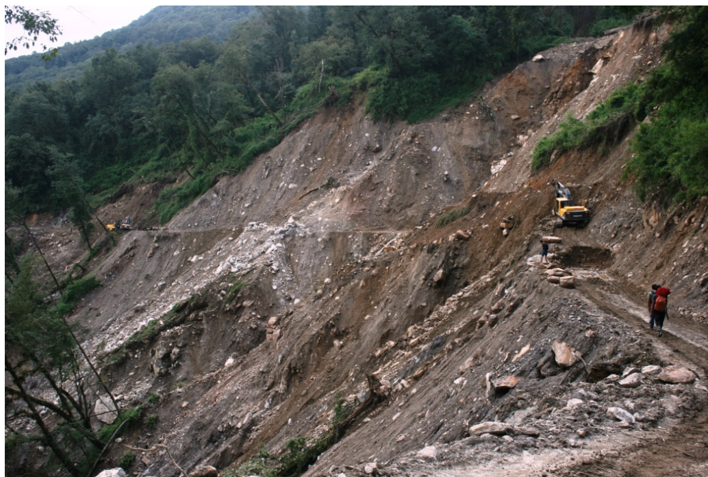
Figure11 The road section close to Damji after the destructive flash floods of June 2012. Multiple road blocks closed the Gasa road for about 3 months, complicating supply and access for the project.
