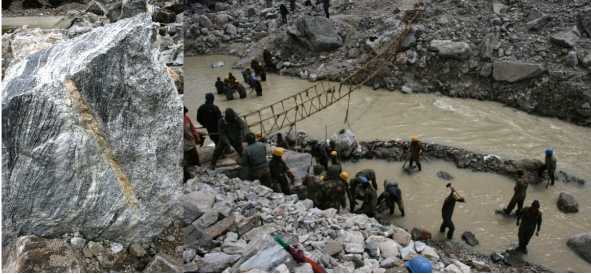
Figure 8 To the left: drilling hole made with a Penjor drilling machine and use of silent explosives to split the boulder; to the right: sub-optimal working conditions near the inlet.
