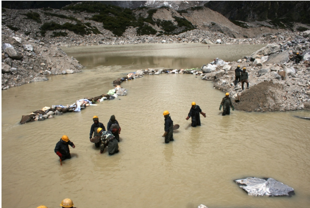
Figure 7 Excavation work near the inlet where an ice lens complicates the work conditions considerably. The workers are part of the 123 RBA personnel.
