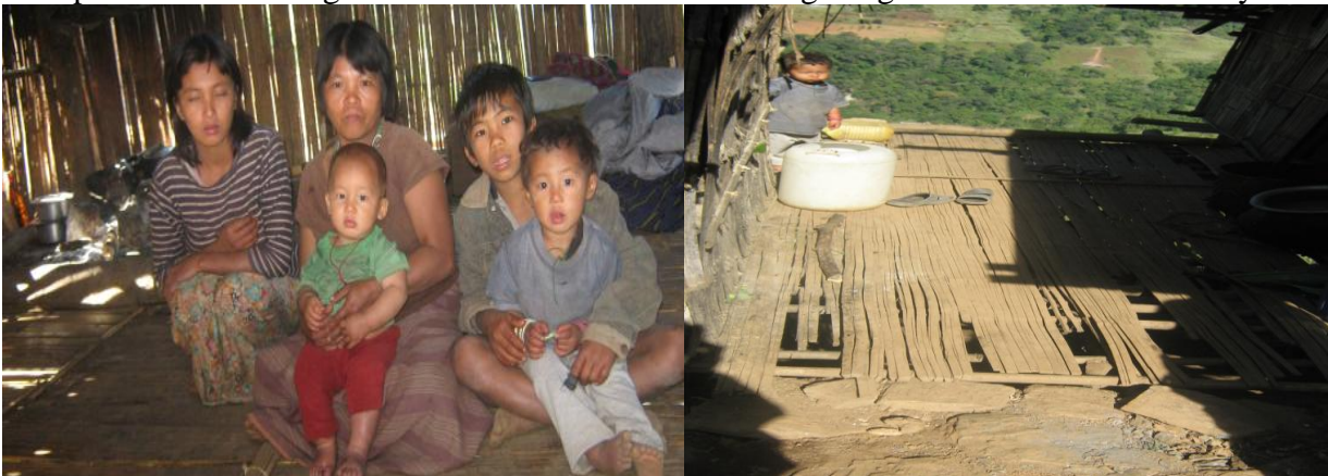
Figure 38: A family inside its dilapidated hut with transparent bamboo railings. A mother of two children (extreme left) prays for a new house while her son cannot negotiate the fragile worn-out door steps. The family now produces its own vegetables and food; the Foundation is also helping the family with construction of new house “which will have a good window through which the family will proudly look out at the world” said the mother of the children. The family estimates that it consumes about Nu.300 worth of vegetables from its new kitchen garden. Like other households, the family planted oranges, arecanut and mango seedlings on Kamzhing .
