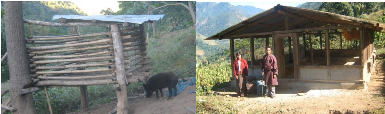
Figure 22: Every household has constructed pigsty with CGI sheets supplied by the Project. All households in the village are divided into two poultry rearing groups; each group has constructed its own poultry shed (right). The group members were given training in poultry management. Piglets and chickens are yet to be supplied by Project.
