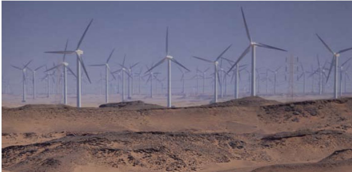
Egypt. The Zafarana Wind Power Plant Project is part of an approach to support national initiatives in promoting a greener economy and the use of renewable energy. © UNFCCC, 2010 C. Anagnostopoulos
