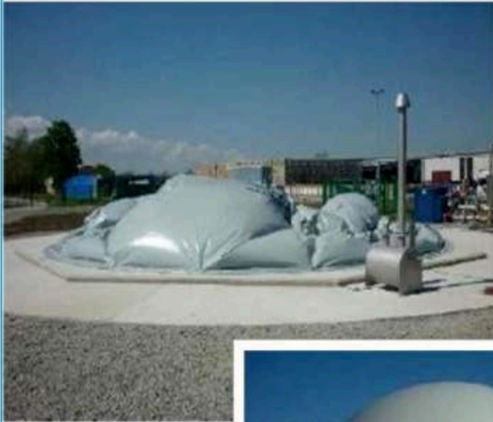
Figure 54 : Flexible gasholder and compressor– Source (GtS) Storage systems can be classified in three main types depending on the pressure.
