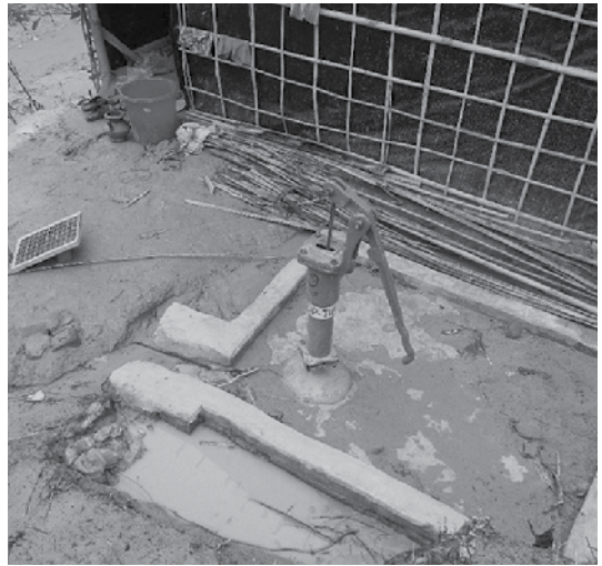
Water well in Kutupalong camp | Photo A.Chaikine, UNDP
