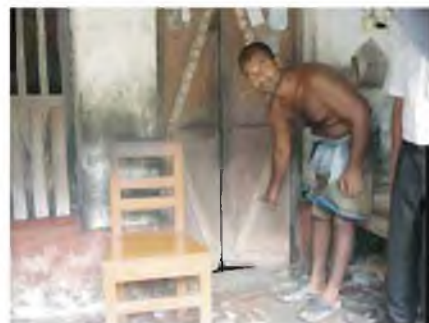
HHs Inundation level due to water logging
