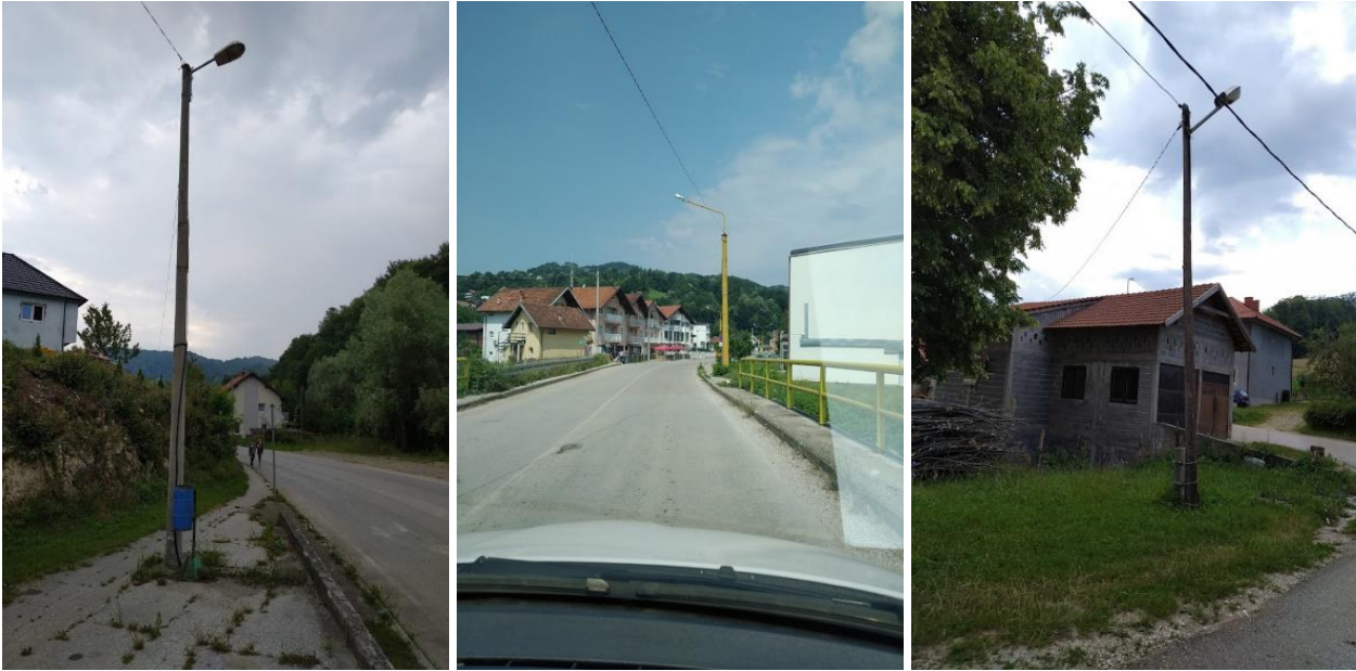
Image 26: Poles (Reinforced concrete - left, metal –middle, wooden-right)
