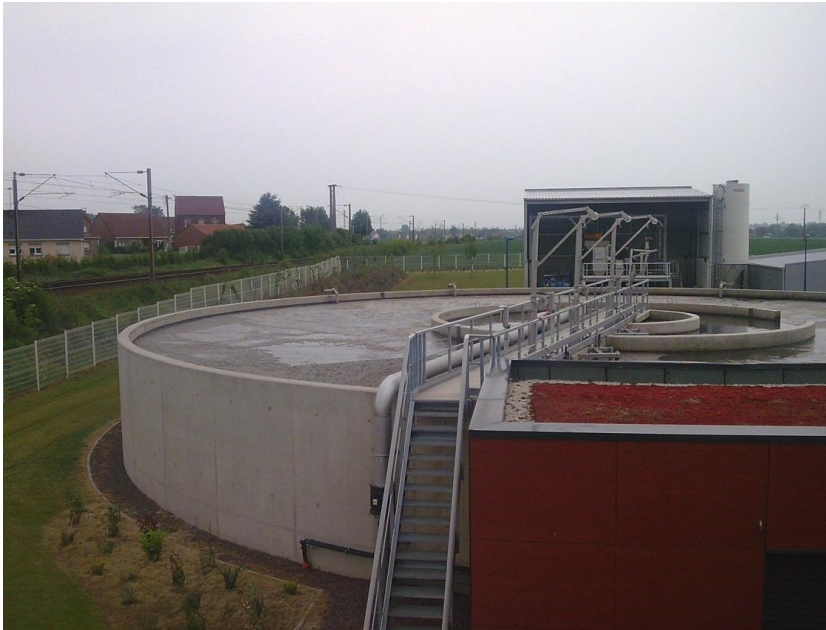
Figure 5.2 Wastewater Treatment Plant Near Lille, France
