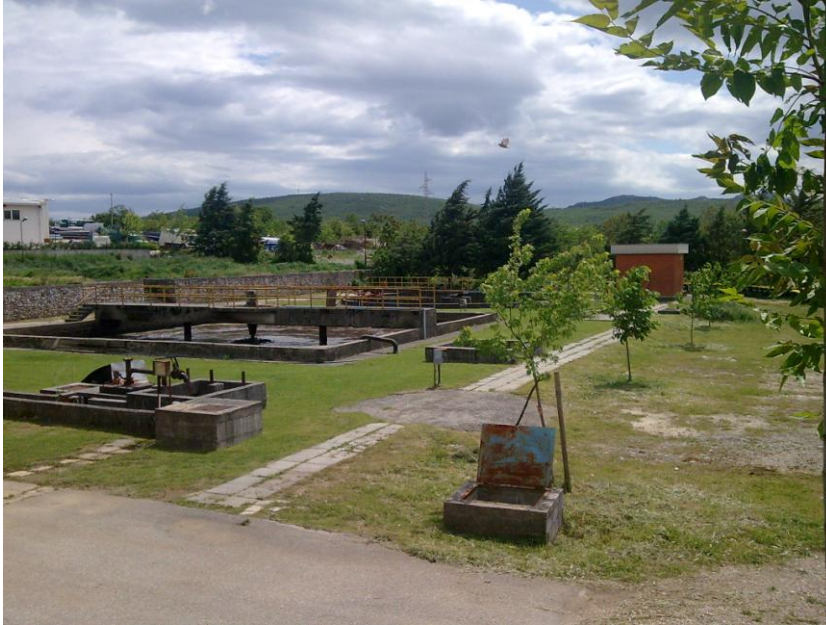
Figure 5.3 Wastewater Treatment Plant in Ljubuški, BiH
