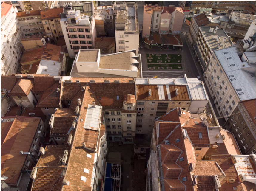
Figure 76. Urban room No. 3: Maršala Tita interior courtyard aerial photos.
