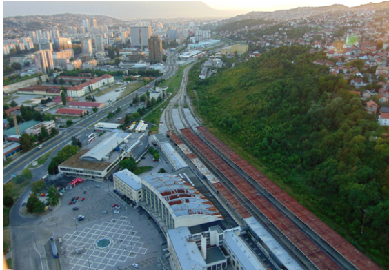
Figure 18. Top: Railway station. Centre: Radio and television headquarters. Bottom: Old electrical power plant.
