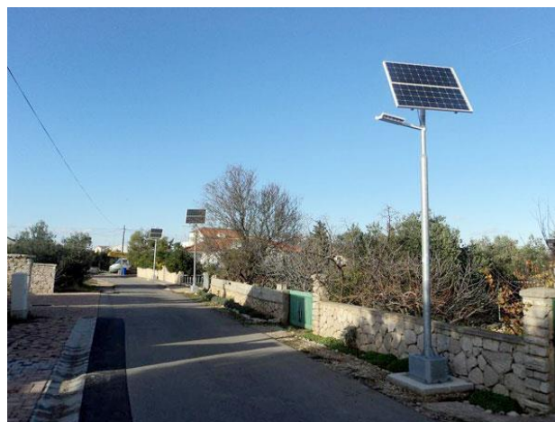
Image 18: Example of solar LED public lighting (island of Murter – croatia)
