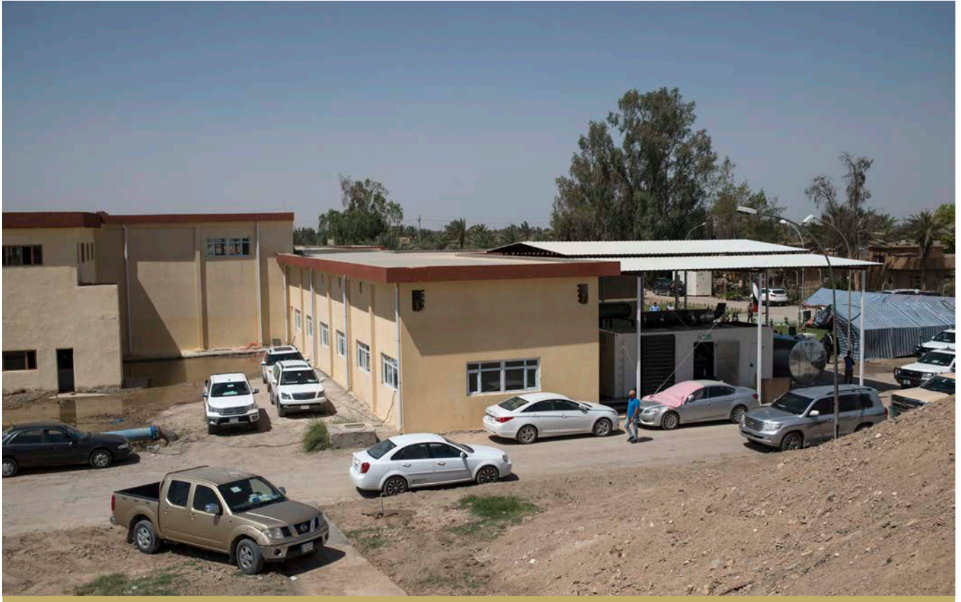
AL AZRAKIYAH WATER TREATMENT PLANT AFTER REHABILITATION IN MAY 2017. © UNDP IRAQ / LINDSAY MACKENZIE
