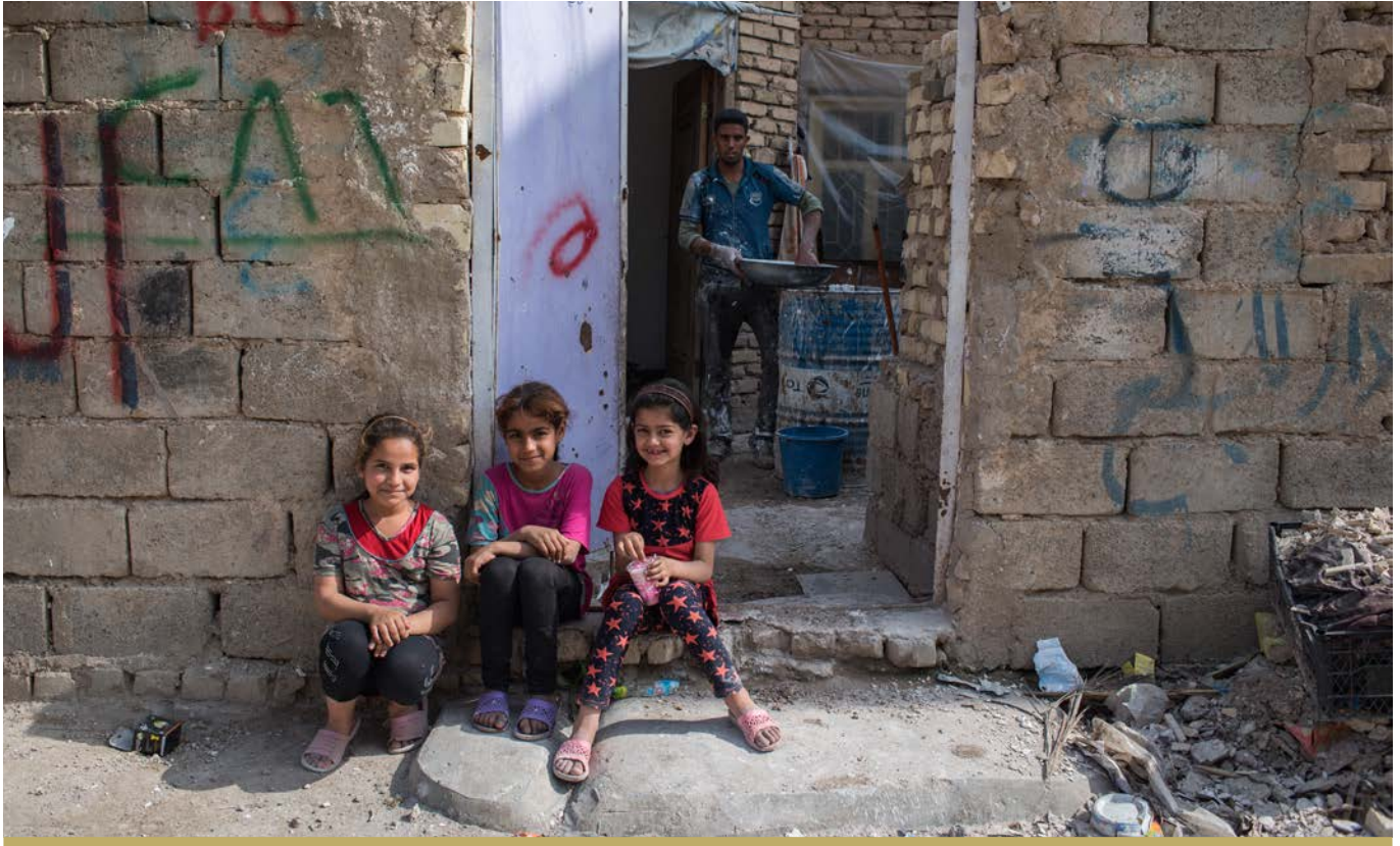
CHILDREN SIT OUTSIDE A HOME WHERE HOUSING REPAIRS ARE TAKING PLACE AS PART OF THE HOUSING REHABILITATION PILOT PROJECT IN FALLUJAH. © UNDP IRAQ / LINDSAY MACKENZIE
