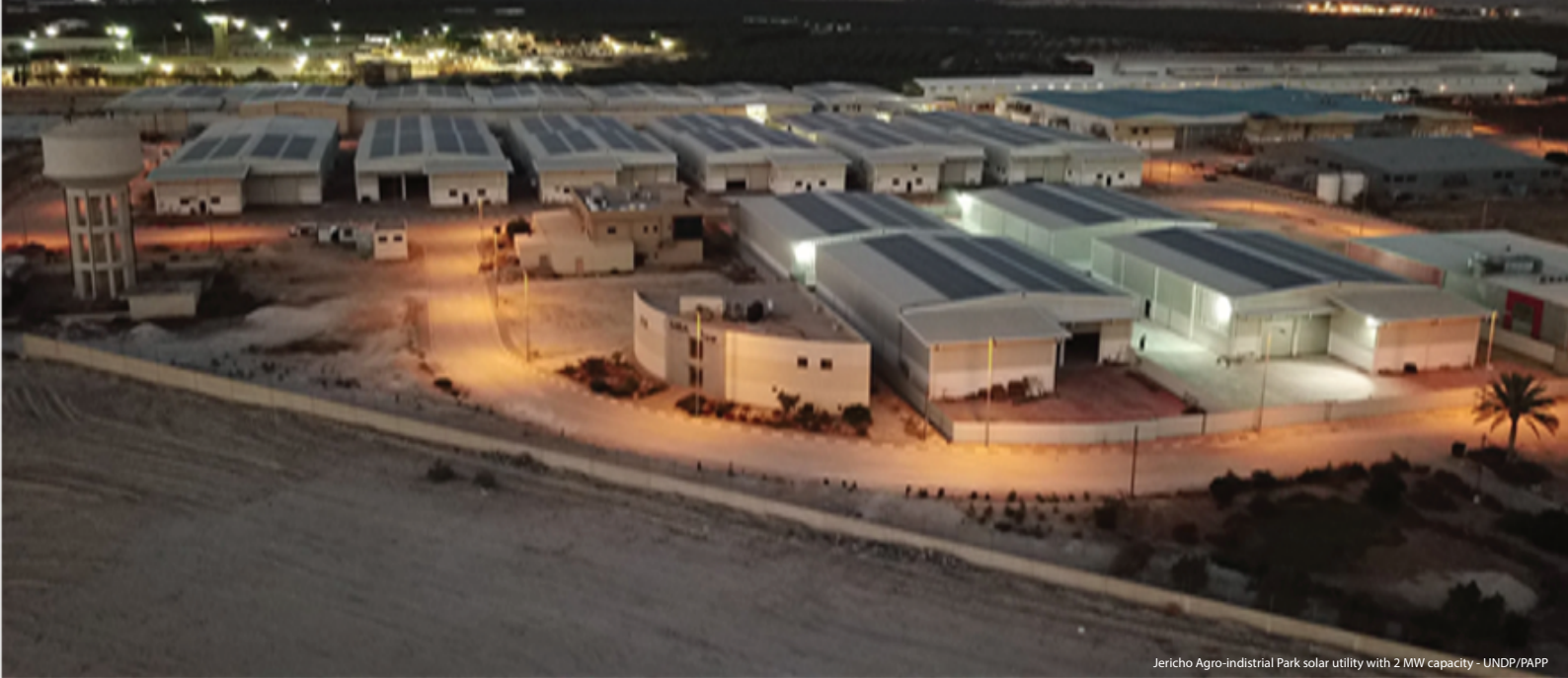
Jericho Agro-industrial Park solar utility with 2 MW capacity - UNDP/PAPP
