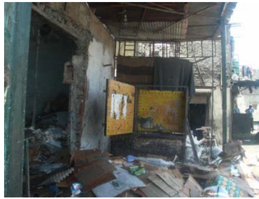
Figure 4.31 Storage area/warehouse of one of the dealers in Gharbia
